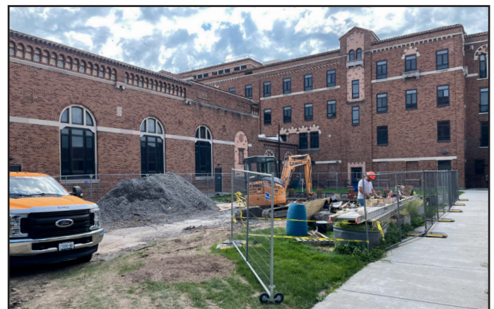
Construction Begins On Enclosed Courtyard Pavilion
